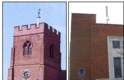
Listed buildings: (1) Antennas disguised as weathervane (2) Poorly sited antennas
