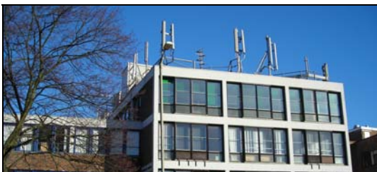
Camouflage: (1) & (2) Antennas disguised to blend in with building features (source: Stappard Howes, Chertsey., Surrey) (3) Overly prominent or multiple antennas detract from streetscene (Summertown, Oxford)
